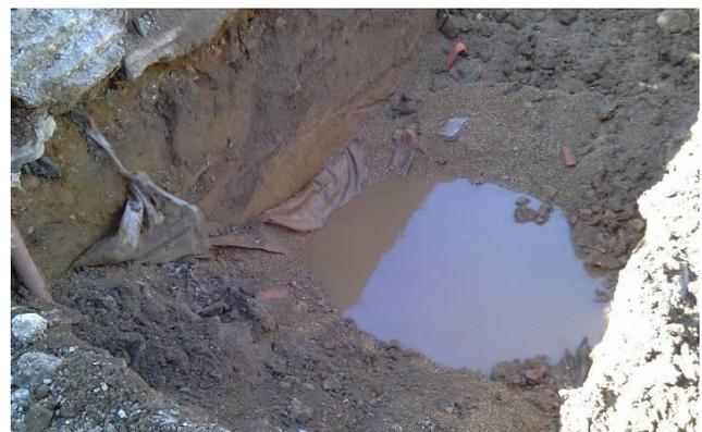
Enviro-treat were able to pump out the liquid tank contents and incorporate into the treatment process. All the tanks were subsequently excavated, cleaned and removed for offsite disposal. The cement slurry filled tanks were emptied and the contents were treated.
