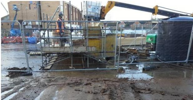
The permeable reactive barrier was installed along the northern and eastern boundaries of the site – the barrier was designed to intercept and treat the natural flow of groundwater migrating from the site with the aim of protecting the prime controlled water receptor (the River Rea) from the risk of pollution from residual groundwater contamination associated with the site as a whole.
