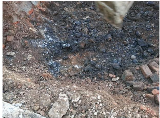
The excavated materials were treated by E-Clay Stabilisation and reused on-site following successful validation - the treated materials were redeposited within the voids created by the excavations.
