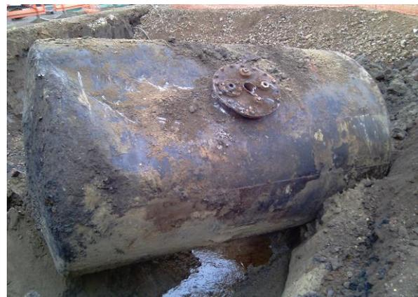
The remaining tank (a 27,000 litre cement slurry filled petrol tank) was left *in-situ*. This was considered necessary due to the tank location being in close proximity to adjoining properties with the perceived risk of structural damage resulting from tank excavation. Enviro-treat were able to demonstrate (through a combination of trial pit excavation / validation and exposing / treating the tank contents as necessary) that the tank would not pose a risk to the future development of the site.
