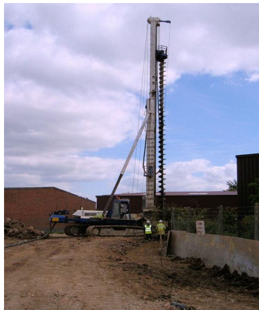
Figure 3 – Barrier Installation Using CFA Auger
