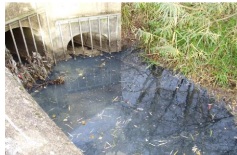
Figure 2 – Surface Water Contamination
