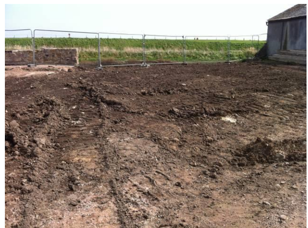
Figure 3 – Site Post Remediation (looking east)
