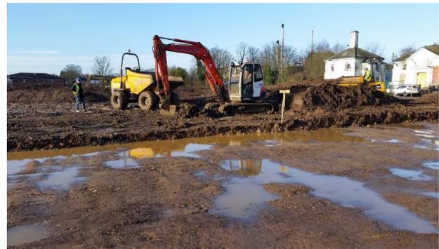
The enabling works included a requirement to carry out an extensive reduced dig to accommodate the foundations and drainage channels etc. The excavation of the foundations for the Sports Hall is shown in Figure 4 below.
