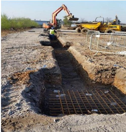
Figure 5 – Excavation of the Attenuation Tank / Underlying Natural Soils
