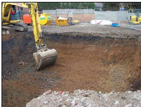
**Plate 2** Excavation of contaminated soils
