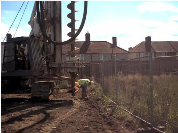
Figure 2. Installing the barrier using continuous auger piling.
