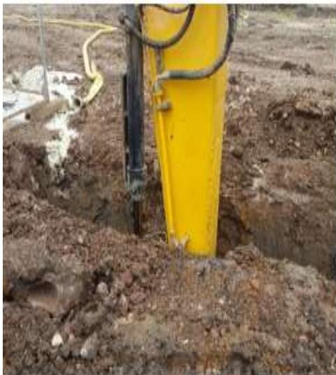
Figure 8 – PRB Installation - Soil Mixing
