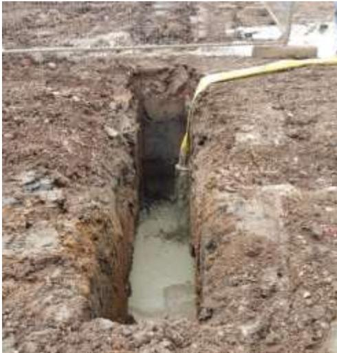
Figure 7 – PRB Installation - Soil Mixing
