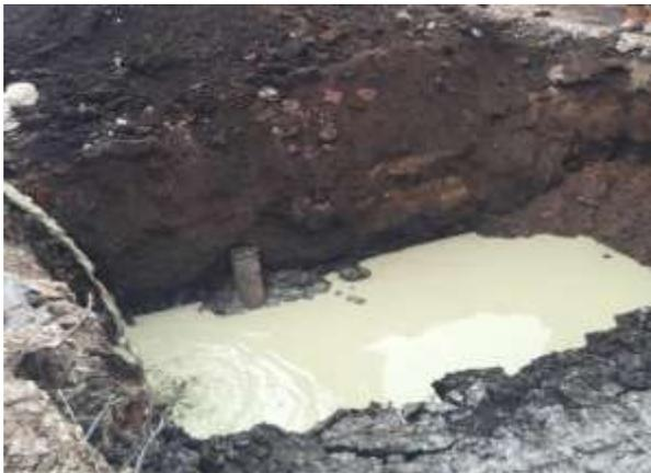
Figure 11 – Source Treatment – Mixing Process
