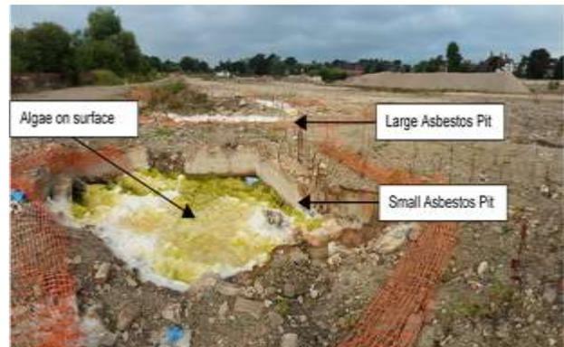
The demolition contractor had previously identified the presence of asbestos contaminated soils and ACM within the machine pits. The ACM contained within the machine pits comprised of cement bound sheeting fragments and insulation board (chrysotile and crocidolite forms of asbestos in the cement board sheeting and chrysotile and amosite forms of asbestos in the insulation board).
