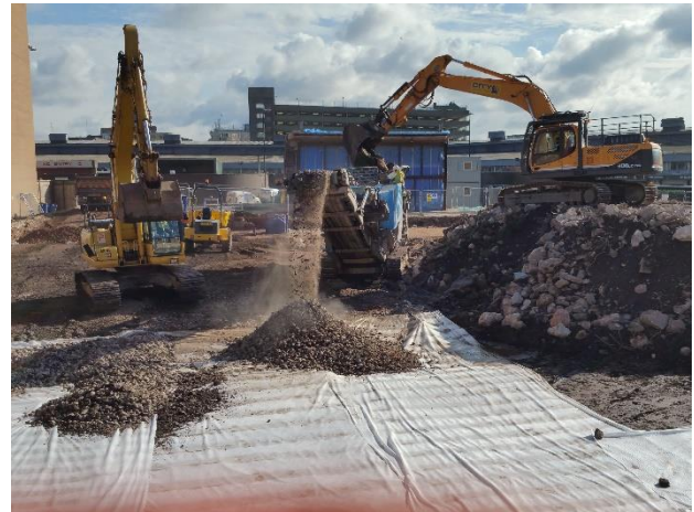
Figure 6 – Provision of piling mat.
