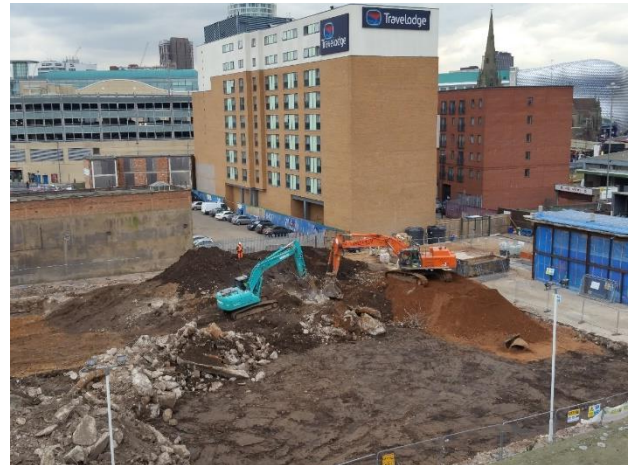
Figure 2 – Photograph showing phased remediation of the Pershore Street Site
