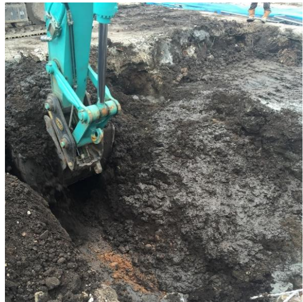
Figure 3 – In-situ E-Clay treatment of heavy metal impacted soils.
