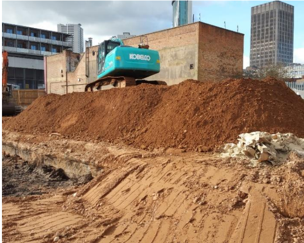
Figure 4 – Stockpiling of natural sands and gravels for subsequent recycling
