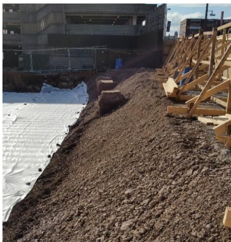
Figure 5 – Temporary works – Batter installed along Pershore Street Side of the Site
