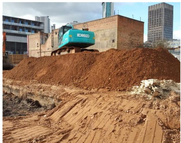
Temporary works were required on the site due to height differences between Pershore Street and development formation levels. Enviro-treat designed and implemented temporary works to remove the surplus soils and replace with a batter comprising of inert soils (designed to be easily removed at a later date).
