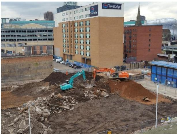
In order to minimise the size of the soil stockpiles being generated around the site (necessary due to site constraints), Enviro-treat treated contaminated soils *in-situ* and removed surplus material offsite as soon as practically possible. There was an implicit requirement to validate the treated soils as soon as practically possible to enable reuse on site.
