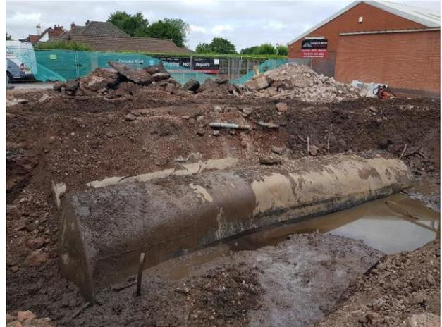
Enviro-treat pumped out the liquid tank contents (water) and incorporated into the treatment process. All the tanks were subsequently excavated, cleaned, tested and removed for offsite disposal.
