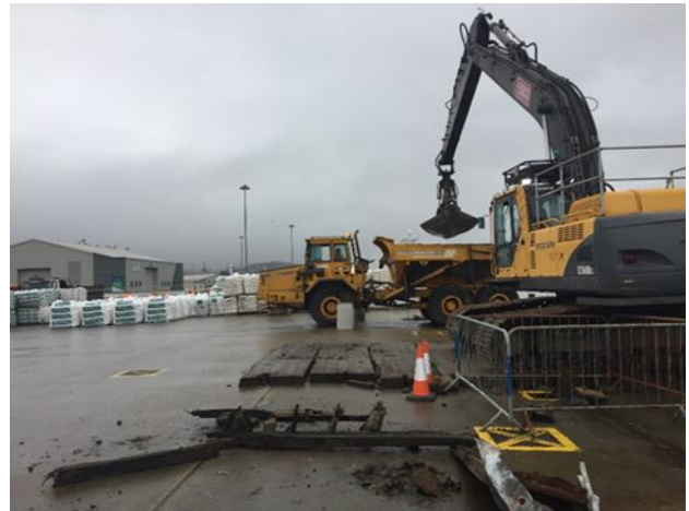
Figure 4 – Loading of Dredged Sediments
