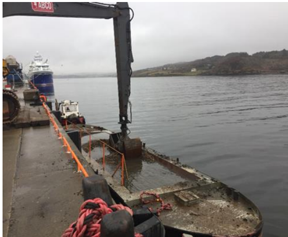
Figure 3 – Offloading of Dredged Sediment
