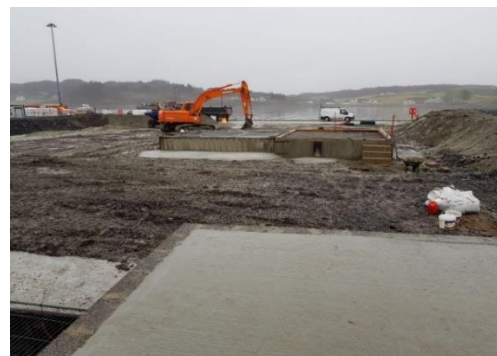
Figure 9 – Construction of Mixing Units
