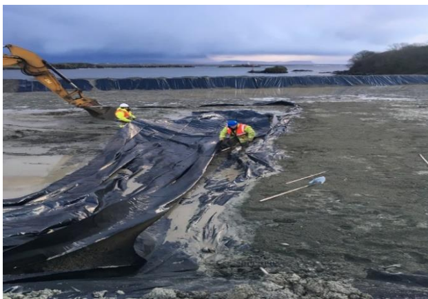
Figure 7 – Installation of Polyethene Lining
