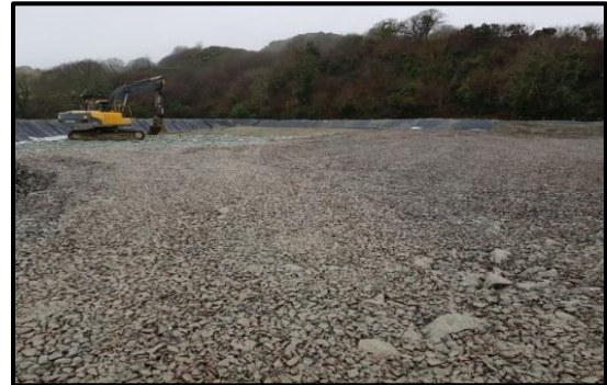
Figure 8 – Completed Treatment Area
