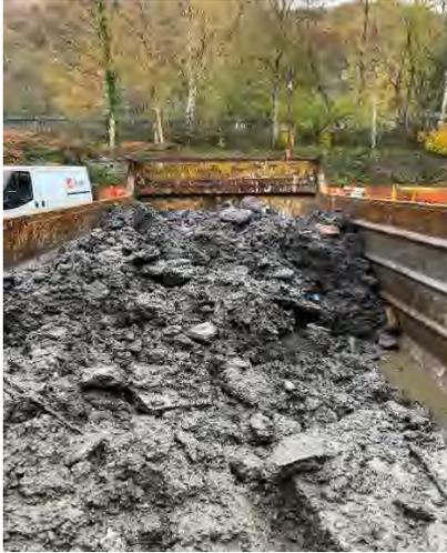
The soils were excavated to the top of the underlying bedrock (circa 1.5 m) and validated by the collection of soil samples at regular intervals from each exposed side of the excavated area. The samples were analysed for TPH-CWG to confirm compliance with the agreed remediation criteria.
