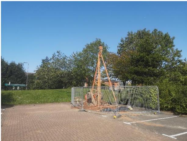
In-situ magnetometer UXO clearance was undertaken in the Made Ground and soft cohesive soils at each location. The provision of stainless-steel lead casing meant that the casing did not have to be adjusted to ensure no interference with the magnetometer.
