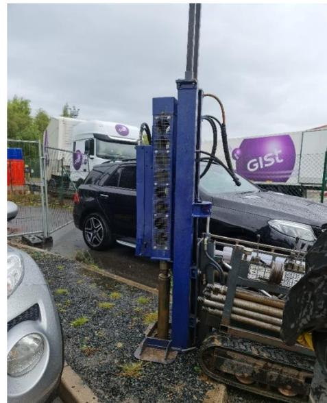
Cable percussion boreholes were advanced using a cable percussion drilling rig at 150mm diameter. The cable percussion drilling is shown in Figure 4 below.
