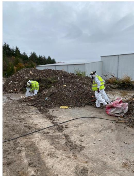
All bagged asbestos fragments were placed in a lined skip for disposal at a suitably licensed receiver site – this is shown in Figure 6 below.
