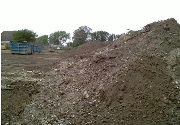
Given the lack of clear guidance it was decided to adopt a precautionary approach. The treatment process incorporated combined physical and chemical stabilisation.
